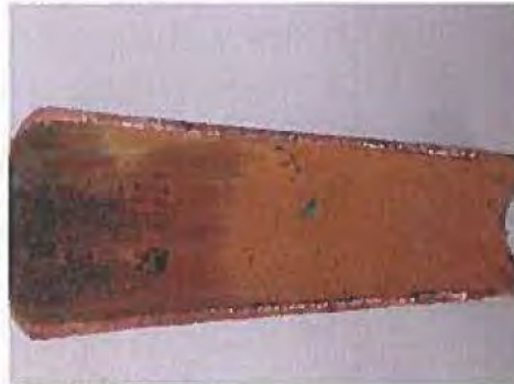
Figure 4-12 Pipe Prior to Scale Removal
