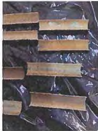
Figure 4-16 Pipes 6A (top 2) and 6B (bottom 2) Prior to Scale Removal
